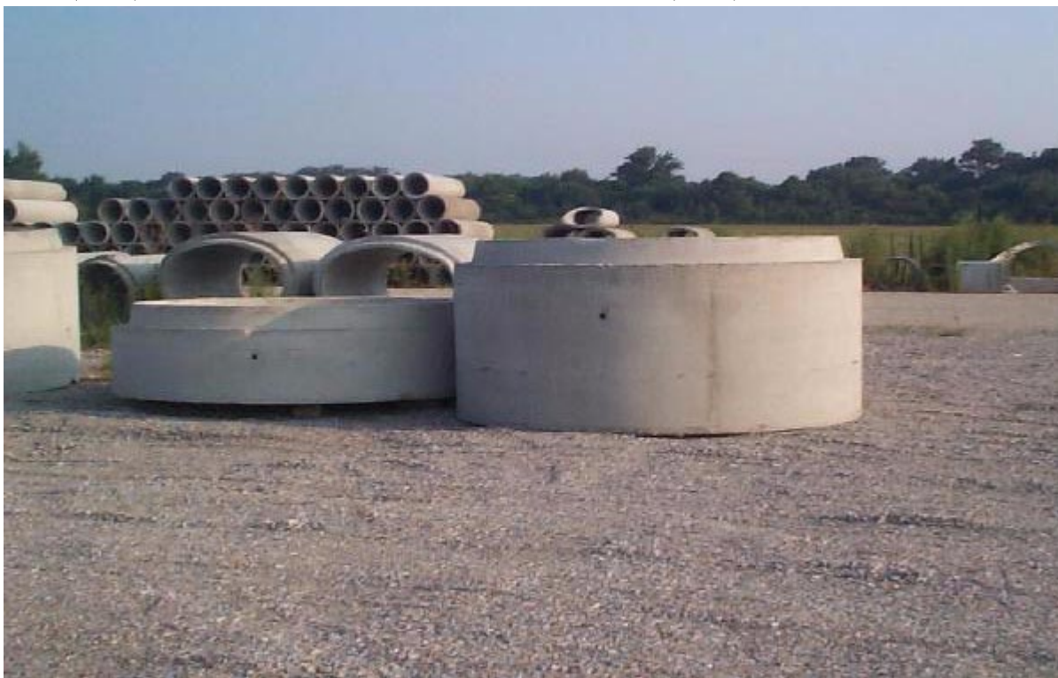
(above) 10' x 10' Precast Wetwell Installation
