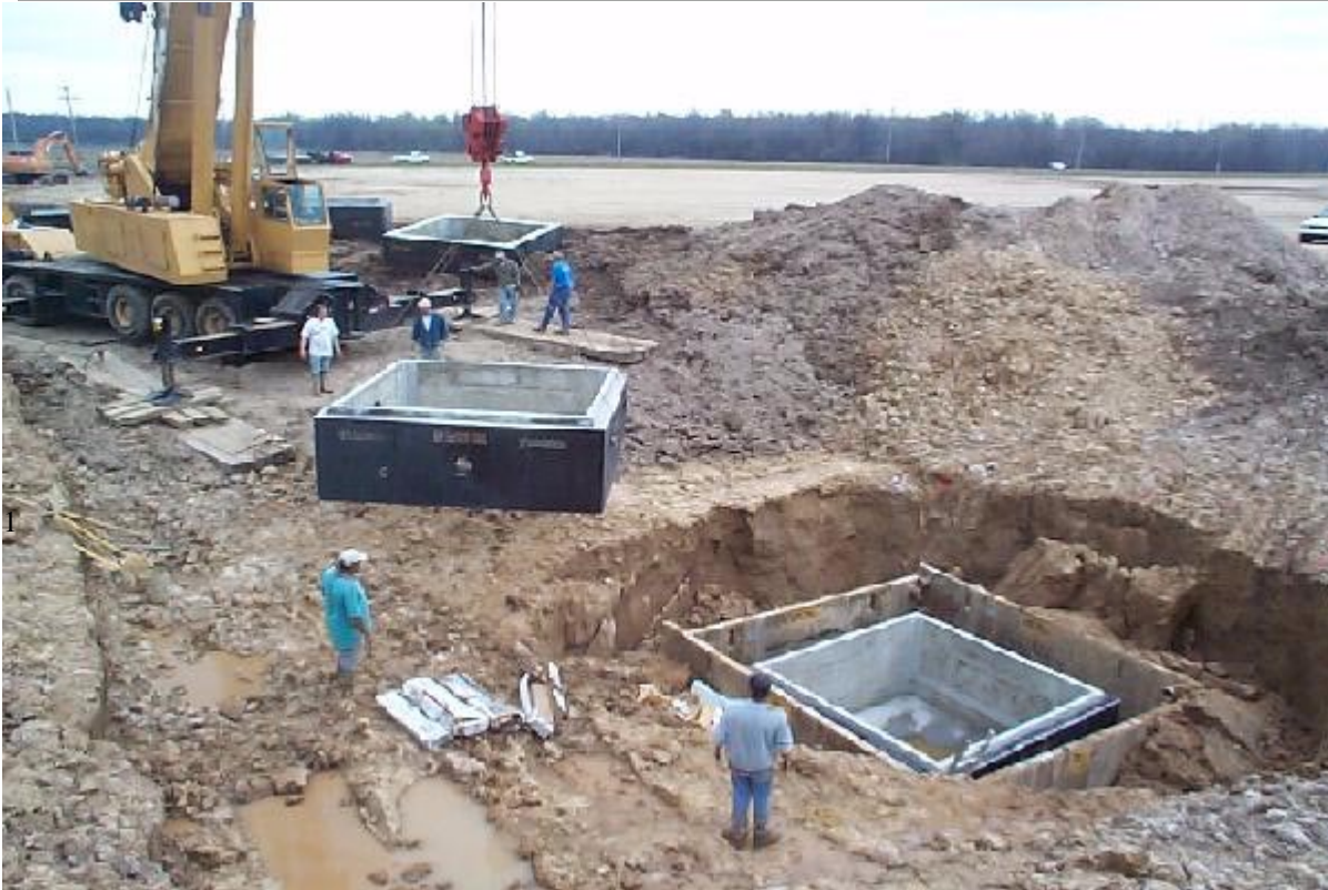
(above) 10' x 10' Precast Wetwell Installation
